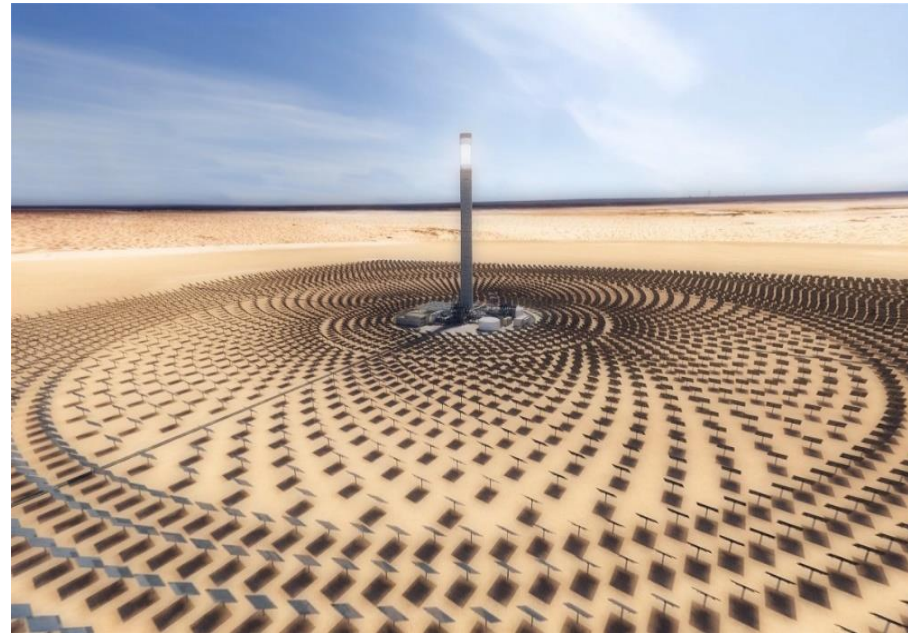
Noor III 510 MW Noor CSP Complex at Ouarzazate, Morocco
